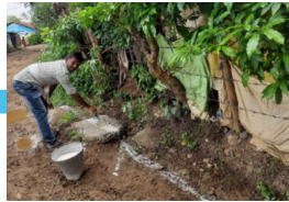
Marking on ground
